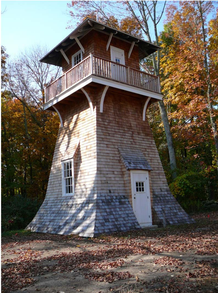
The John Otis water tower built in the late nineteenth century is one of several water towers located in the Town of Norwell. The purpose of the tower was to provide an attractive enclosure around a storage tank supported thirty feet above ground which supplies water on an as-needed basis by a gravity system, distributing water around the property.
